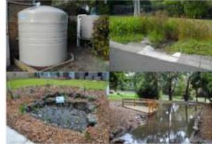
Examples of stormwater control measures installed as part of the research (clockwise from top left: residential rainwater harvesting tanks; roadside infiltration basin; large scale infiltration basin; and residential rain garden).
